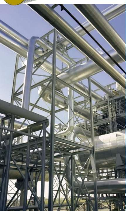
Tru-Roc 1200 Pipe Insulation is produced from the industry's highest quality stone wool. Our pipe covering products can be used up to 1200° F (650° C) per ASTM C447 for use on High Temperature pipes used in the power and petro-chemical systems.
